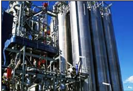
Crane cable lubricants dry out, trap dirt and fail to prevent corrosion after 12 months.
